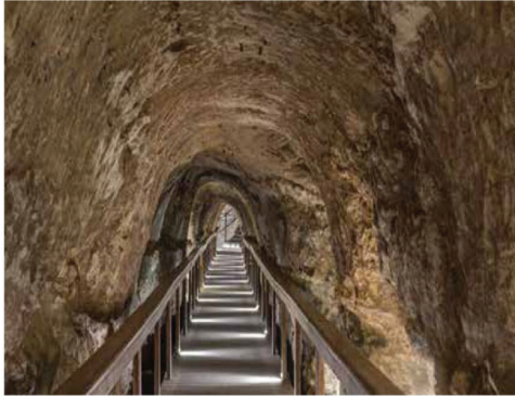
Photo # 5 — The water tunnel cut through rock under Tel Megiddo tapped into a hidden underground spring outside the walls, funneling the water back into a deep cistern within the walls.
